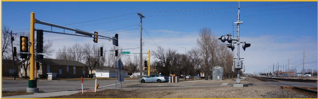
20th Street South Intersection, Facing North
