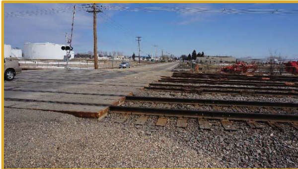
BNSF RR Crossing east of 20 th Street
