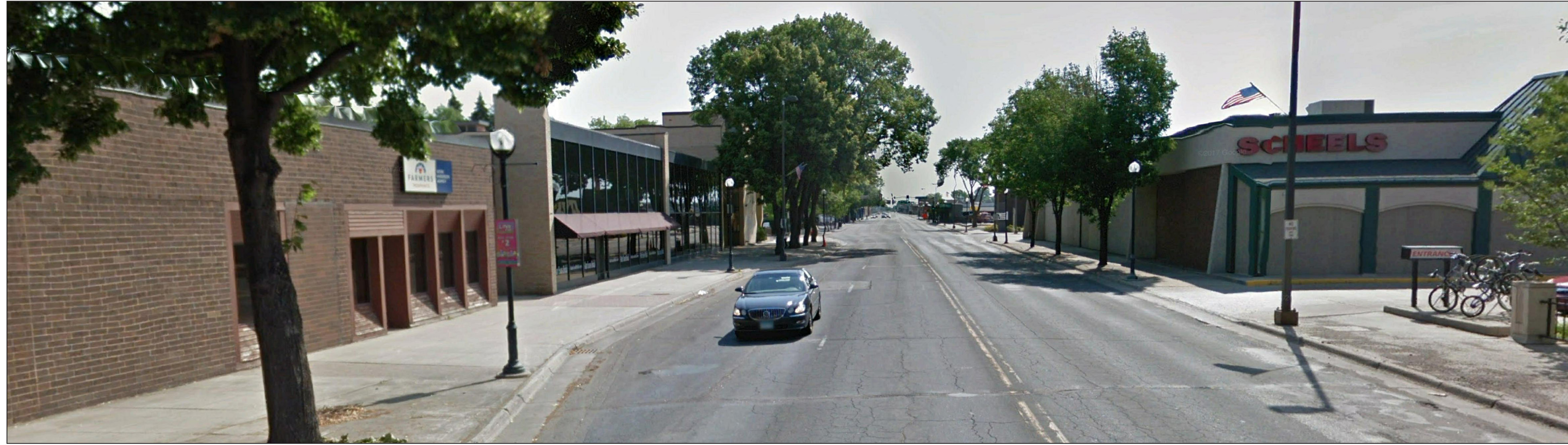
Existing Conditions of Center Avenue at 5th Street Looking East
