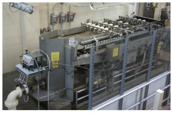
the large sludge particles are scraped off. Thickening improves the performance of the anaerobic digesters and reduces pumping and heating costs.
